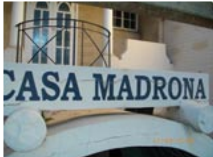
←close-up of existing canopy before repair
