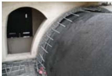
Formwork & doweling in place
