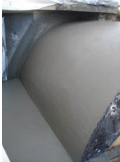
Finishing off the concrete
