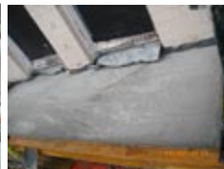
Left: Walls rebuilt and stabilised before formwork erected. Right: Concrete mix pumped to balcony sites ready for membrane and tiling
