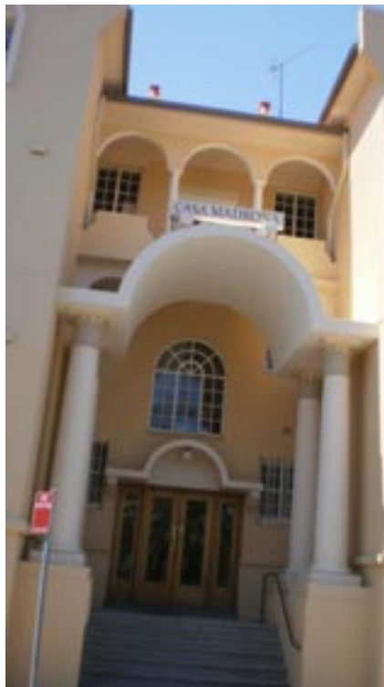
The entrance canopy after being expertly restored and protected
