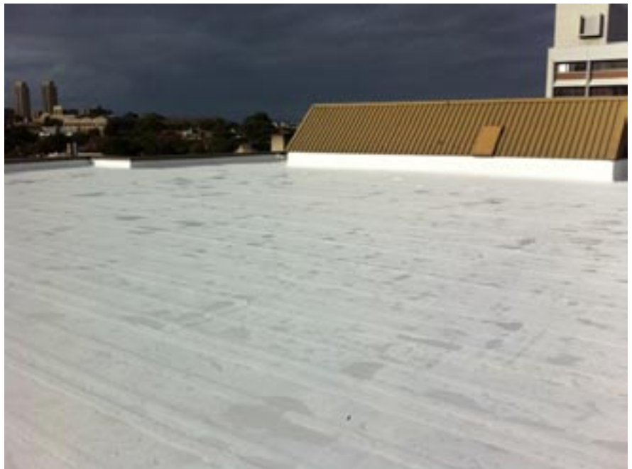
A UV-stable coating was applied
