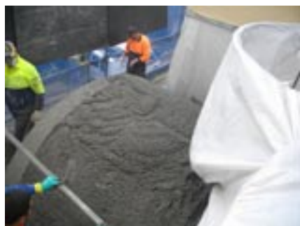
Concrete placed over formwork
