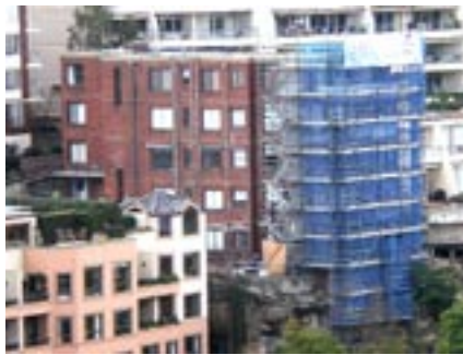
Under way: from Harbour Bridge
