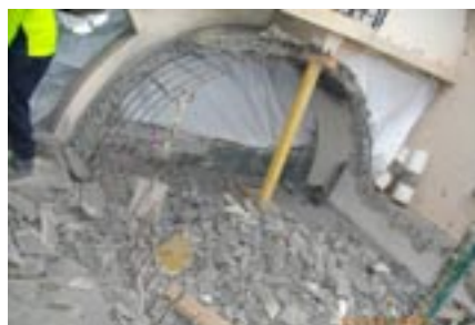
Entrance canopy demolished
