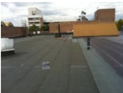
Mineral finish layer installed and detailed
