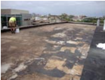
Distinct roof sections stripped, primed and covered
