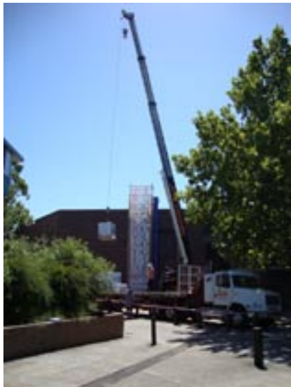
A crane was needed to lift materials to the roof areas
