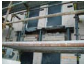
Left: Walls rebuilt and stabilised before formwork erected. Right: Concrete mix pumped to balcony sites ready for membrane and tiling
