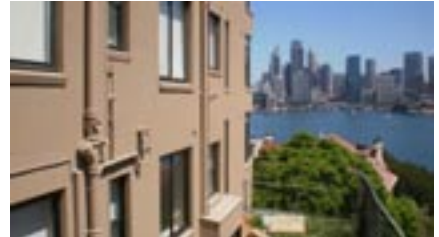
View along West elevation
