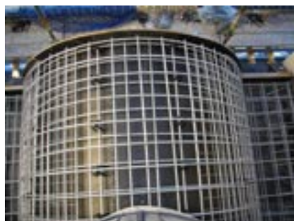
Steel reinforcement in place
