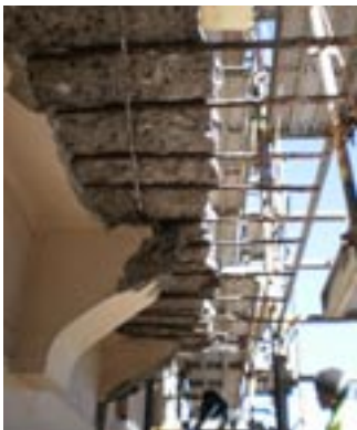
Left: Walls rebuilt and stabilised before formwork erected. Right: Concrete mix pumped to balcony sites ready for membrane and tiling
