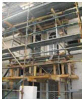
Below: Formwork in place, new steel dowelled in and reinforcement placed
