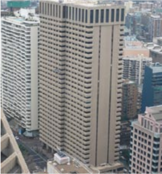
High rise facade repairs need specialist skills by teams experienced in working at height
