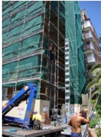
Stage one works to rear tower
