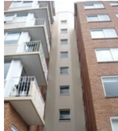
Lift shaft exterior done
