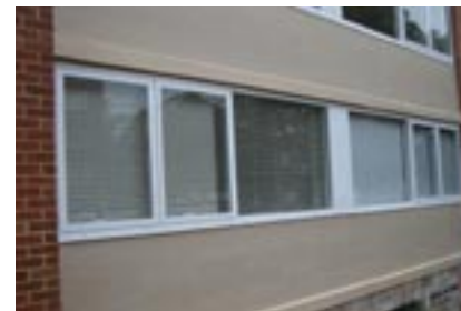
Spandrel tiling and window
