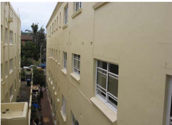
The west elevation approaches completion
