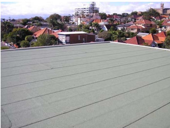
The finished job is attractive and waterproof
