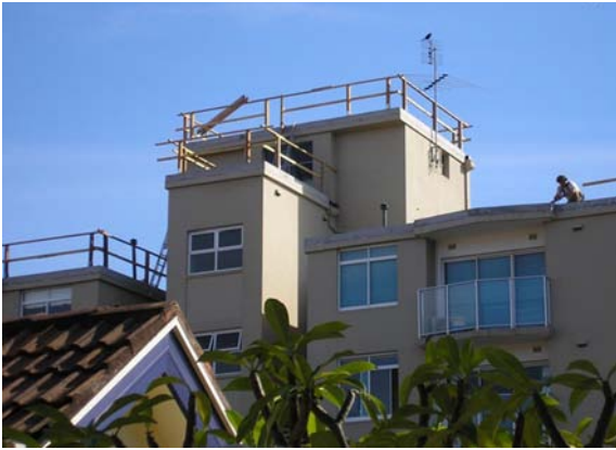
Safety rails are installed in place for Stage 2
