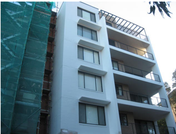
Nearing completion repair and protection
