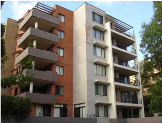
Eddy Avenue elevation prior to repair
