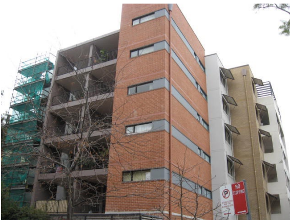
Freeman Road brick facade repointed and cleaned
