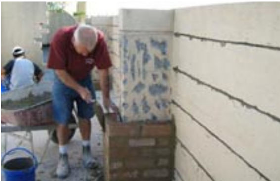
New piers being built and Helifix installed
