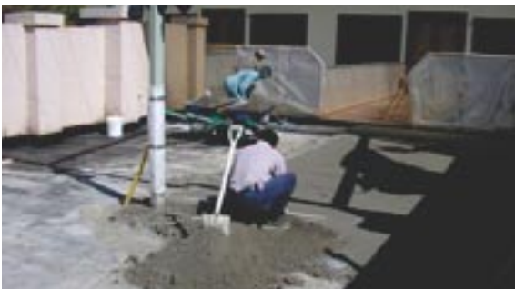
Typical terrace after demolition and installation of the membrane
