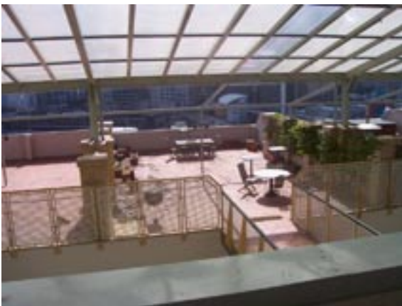
Terraces have been restored and protected
