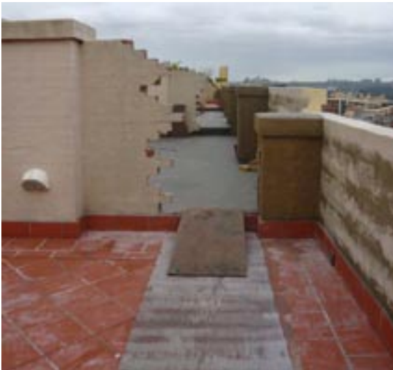
Terraces were opened up for continuous work
