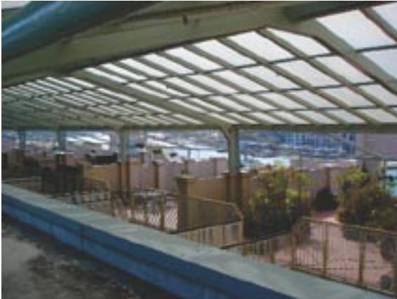
Typical terrace area shows a dividing wall and parapet wall
