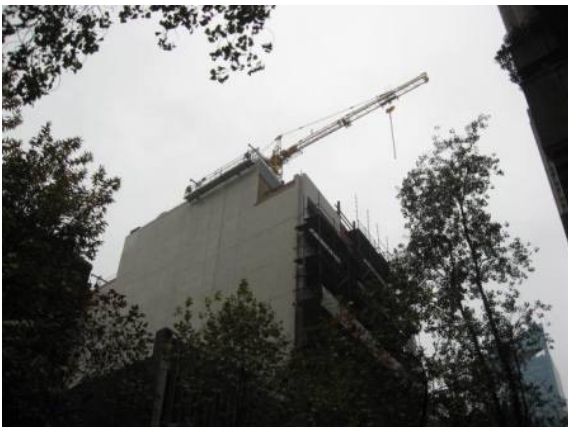
Southern facade repaired and coated
