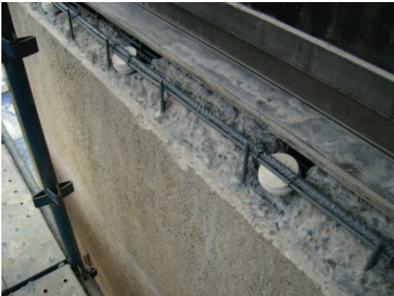
Sacrificial anodes in window sill ready for repair
