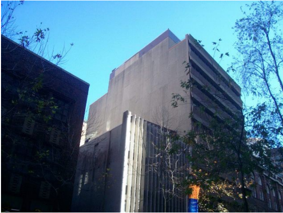
Southern facade prior to protection
