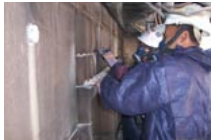
Removal of contaminated mortar
