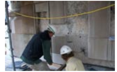
Installing new stonework
