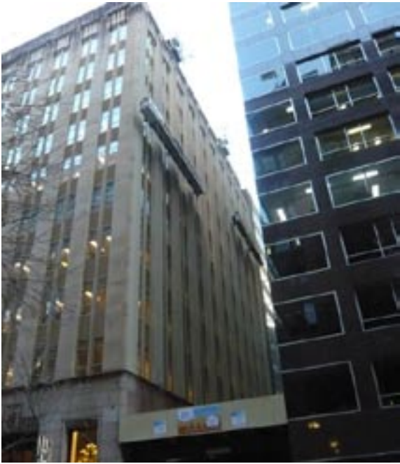
Above: Swing stages over hoardings for investigation, and repairs Below: Crane lowers pavers
