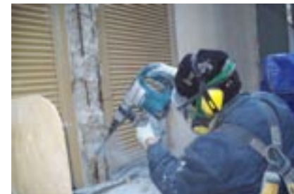
Typical mullion repair detail
