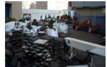
Pavers prepared and removed
