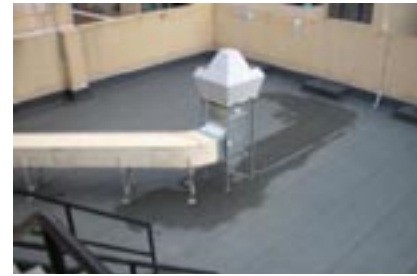
Roof membrane applied to roof
