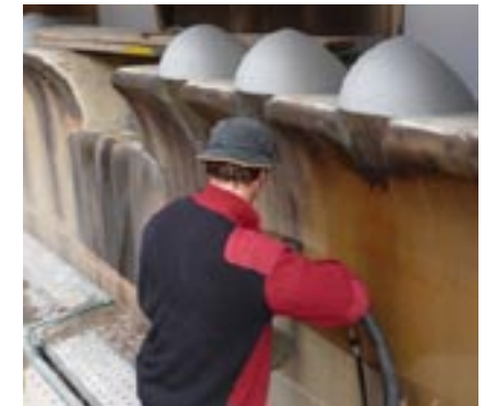
Cleaning stonework to all of the parapet and Level 10
