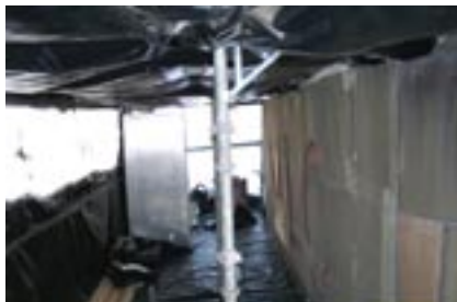
Asbestos removal encapsulation
