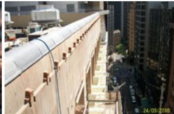
Parapet badly environmentally stained (left) has been repaired, repointed and cleaned with Juliet type balconies waterproofed and protected (right)
