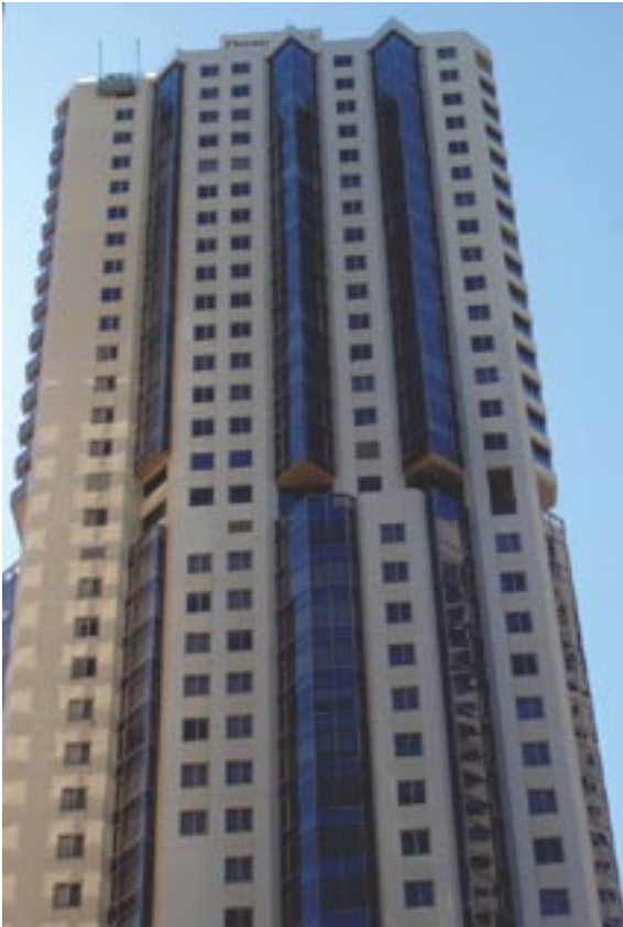
Application of protective coating to western elevation under way
