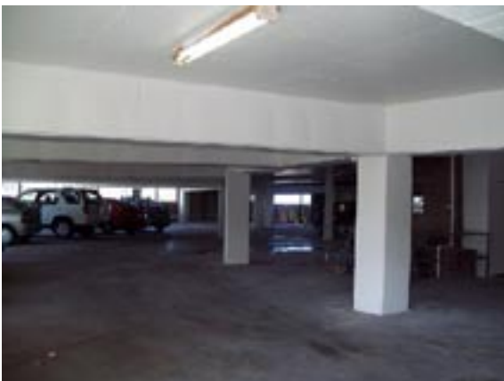
Carpark repairs completed and coating applied
