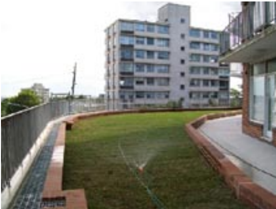
Podium repairs completed
