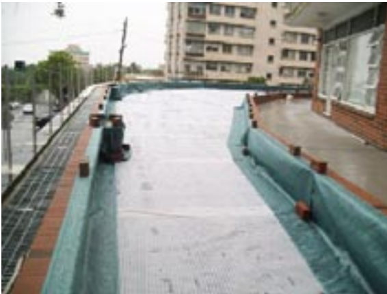
Podium repairs underway
