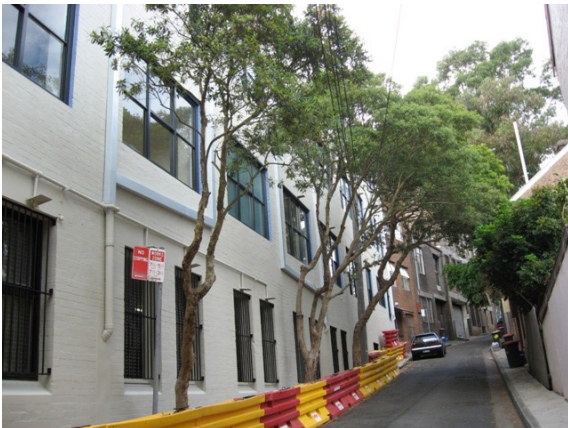
Facade done, with work zone yet to be removed
