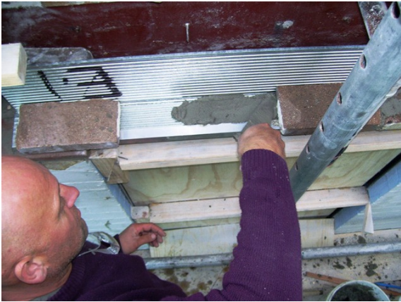
Lintels were built after major prep work internally
