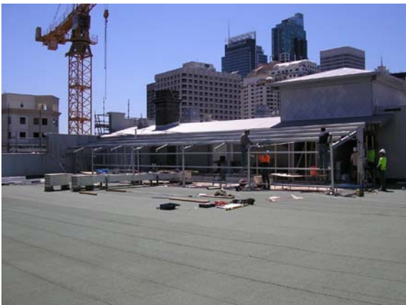
Construction of the new steel structure got under way on schedule
