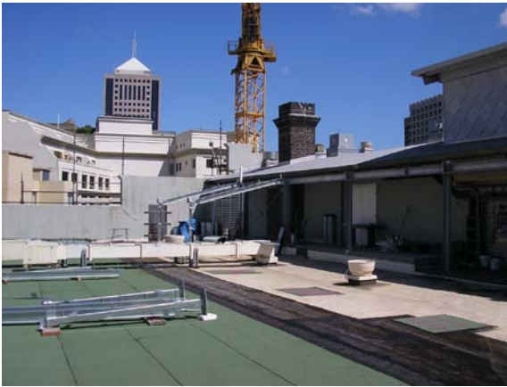
The team laid the new membrane up to the new structure
