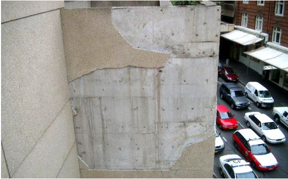
Above: Delaminating render. Below: Safety hoarding also catches repair process water
