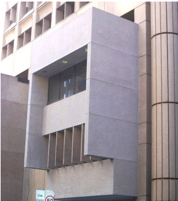
Restored facade area matches existing facade
