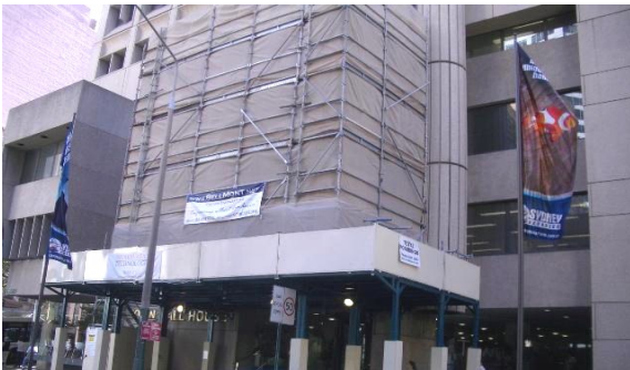
Above: Delaminating render. Below: Safety hoarding also catches repair process water
