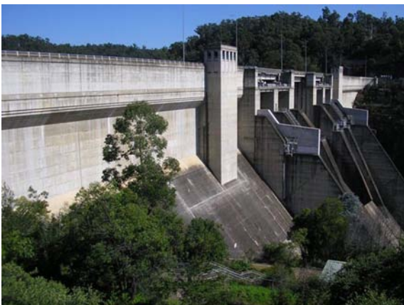
Repairs to the dam wall were completed safely
