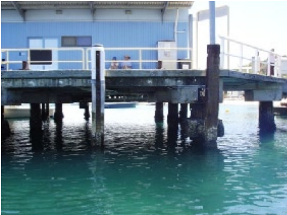
Project overview prior to demolition and repair
