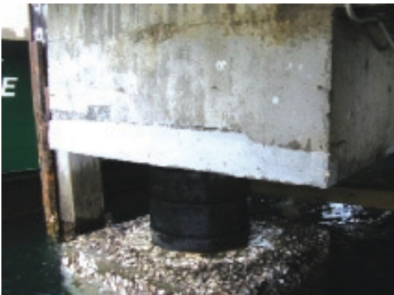
Repair area formed and poured ready to finish off
